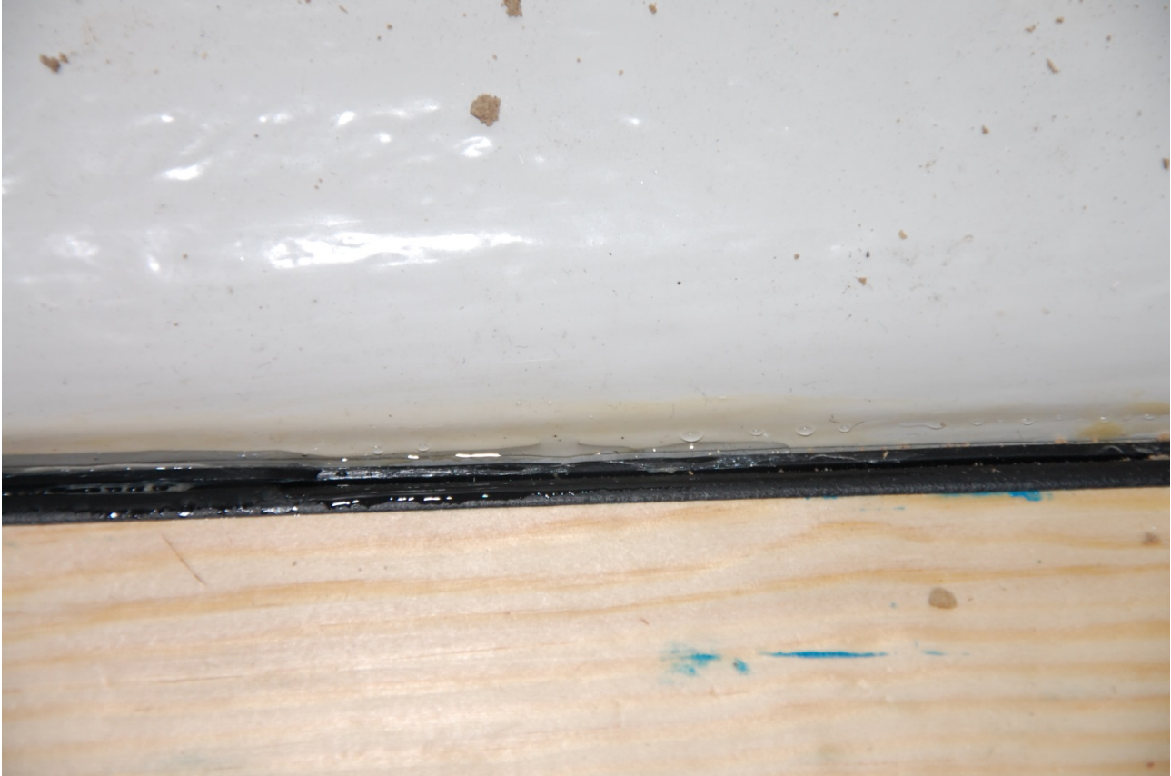
Figure 3.1: Water on seal of product demonstrating low leakage.
